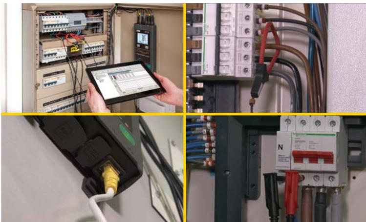
Thankfully nowadays you can purchase a PEL to perform whatever logging you need around the installation, and then semi-permanently and non-intrusively install it in the distribution cabinet for continuous monitoring.
